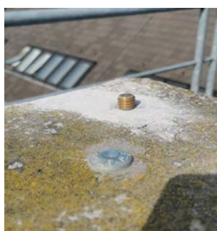
Figure 3. – The top of the pillar
