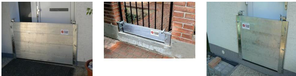
Figure 8. Examples of small metal systems of flood barriers – door protection [11]
