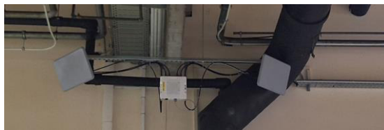
Figure 2. Installing and commissioning the first AP
