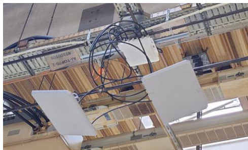
Figure 1. Test device equipped: Cisco IW9167E and two AIR-ANT2513P4M-N dual-band antennas
