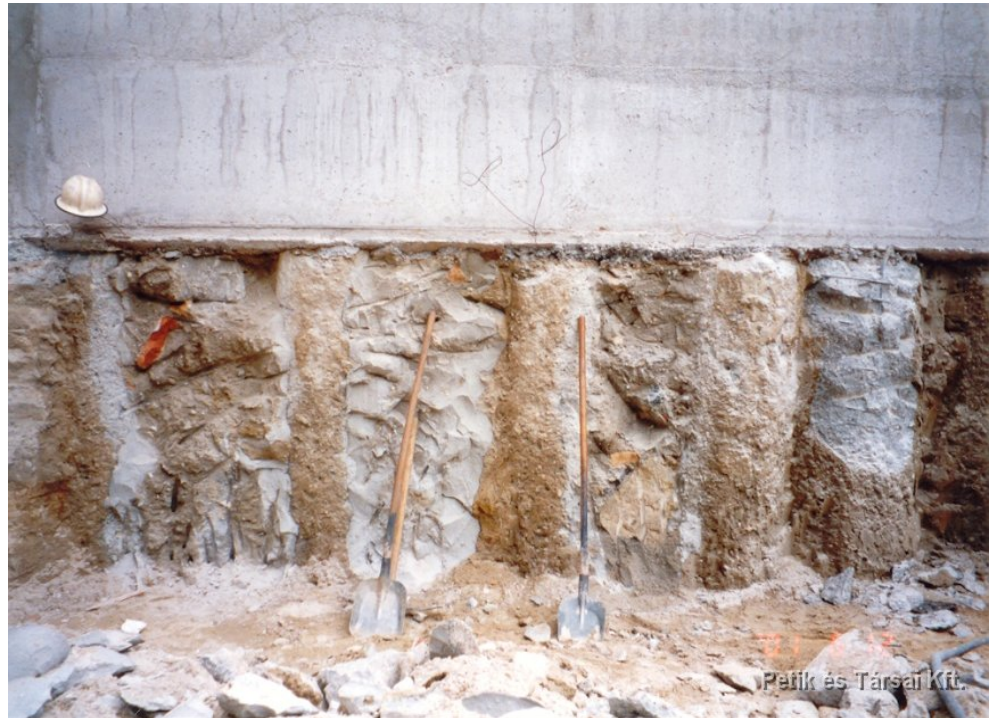
10. ábra Jet-grouting
