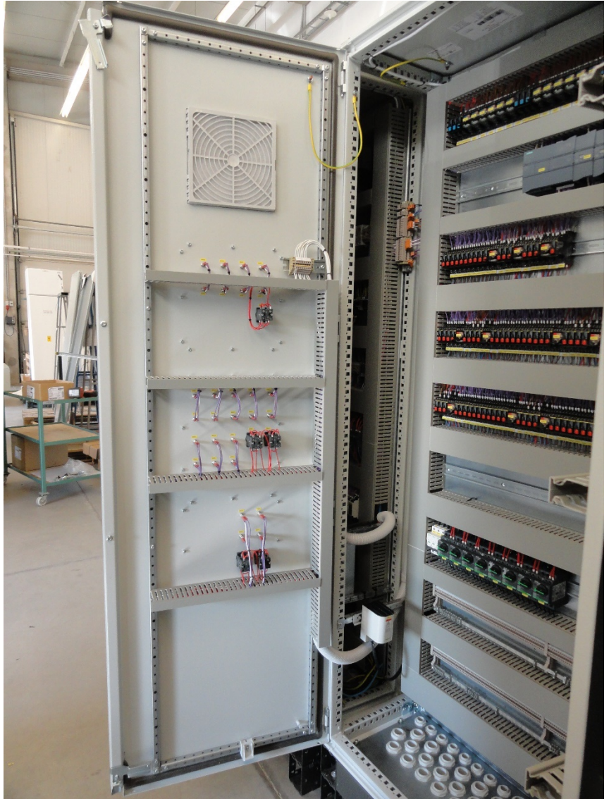
Figure 76 - Internal view of F2 [33]
