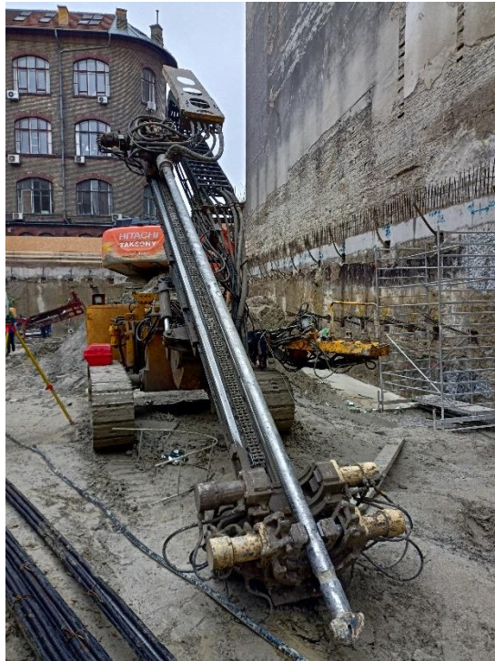
12. ábra Jet-Grouting
