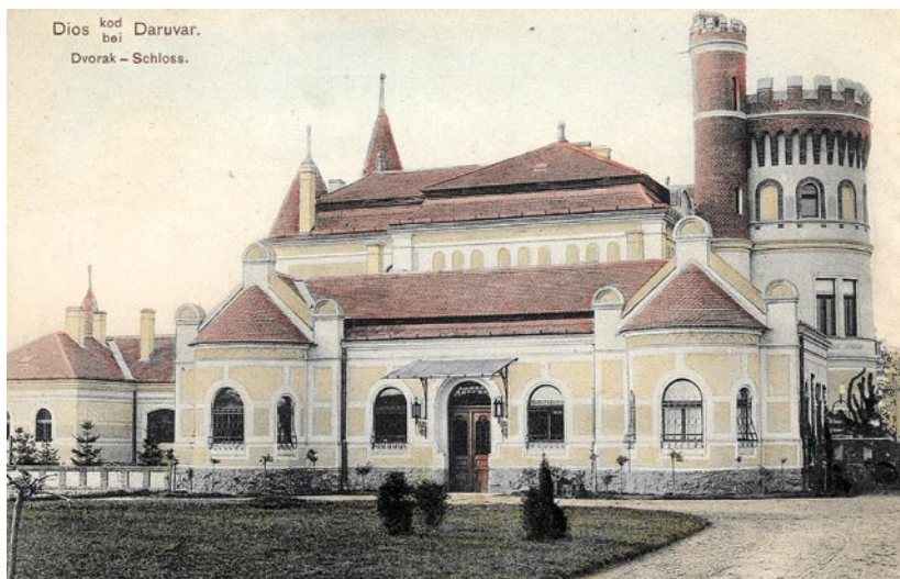
Figure 1. Tüköry Mansion in Dioš around 1910, view from the south [2]
