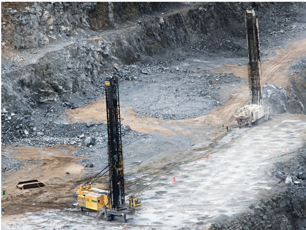
4.4.ábra: Mélyfúrási lyukak létesítése [ https://www.mtu-solutions.com/content/dam/mtu/application/mining/images/04A_MTU_Drilling-in-mining-rigs.jpg/jcr_content/renditions/original/04A_MTU_Drilling-in-mining-rigs.jpg ]
