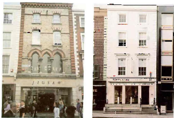
Figure 4: Examples of signage in Dublin that harmonise with the rest of a building. Reproduced from: [20, p. 1, 26] with permission from John O'Hara, Dublin City Council.
