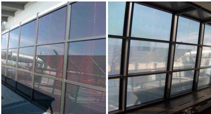
Fig. 1. Thin film solar cells at the glass corridor of Technical College of München, from outside (left) and from inside (right).
