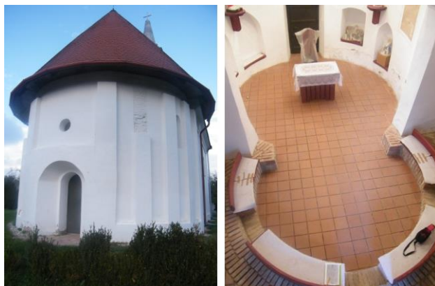
Figure 15. Bagod church outside and inside today
