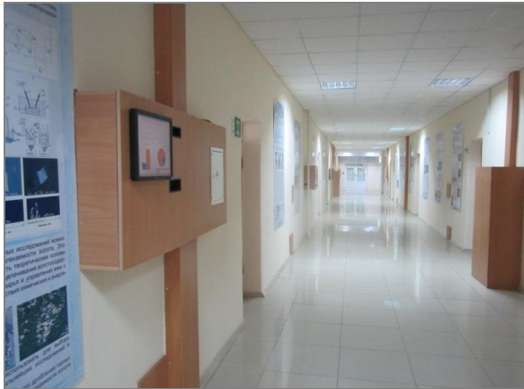
Figure 4. LED lighting of the floor educational building
