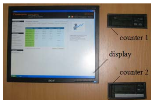
Figure 13. Test bench the electricity consumption over two floors
