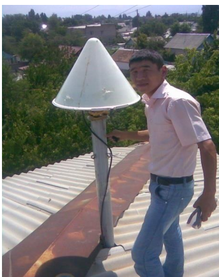
Figure 2. GNSS antenna of KyrPOS CORS [7]
