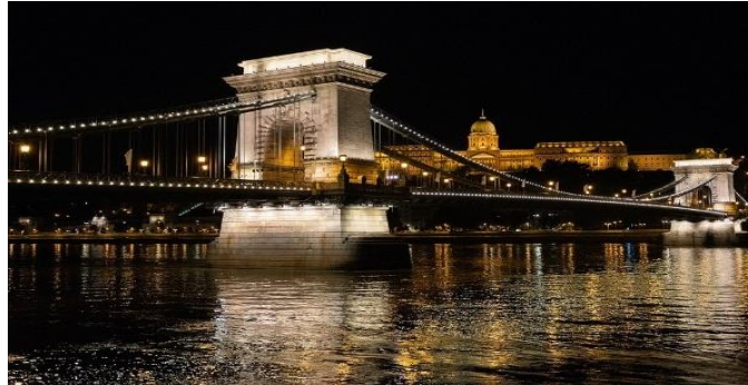
Figure 55: Széchenyi Chain Bridge 125 in Budapest in 2019, before renovation [105]
