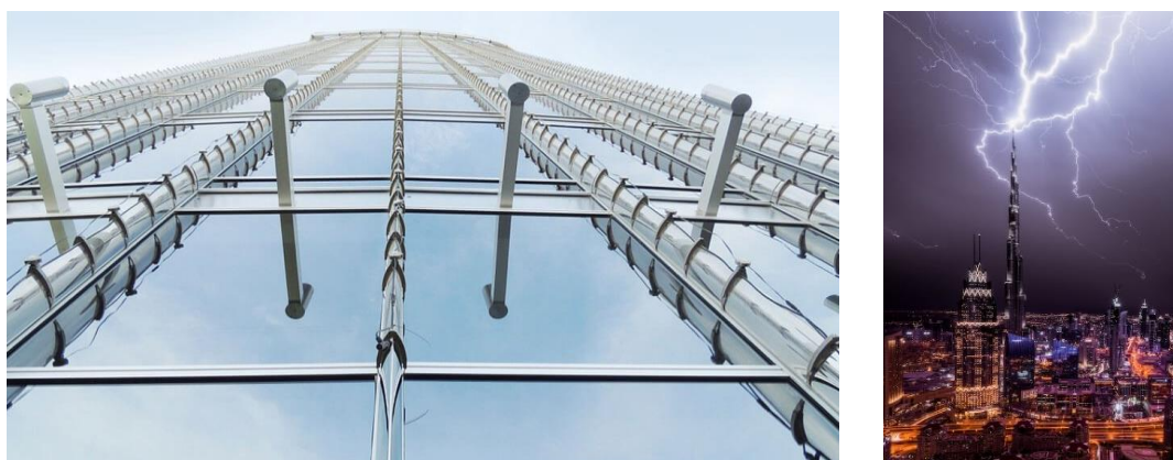
Figure 53: Two pictures of the Burj Khalifa [102] [103] On the left: metal parts of forefront, on the right: during lightning
