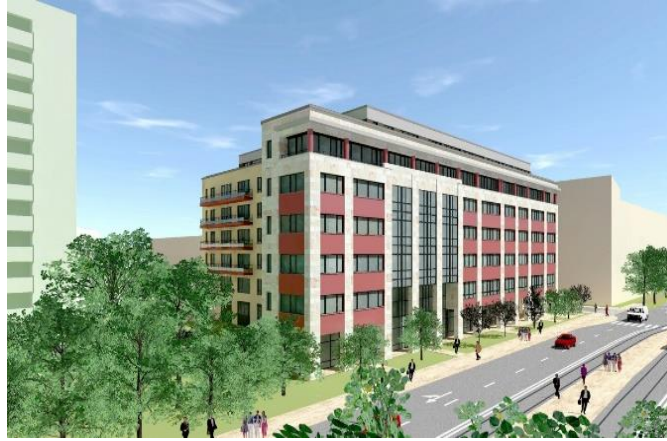
Figure 30: Similar planned office building [58]
