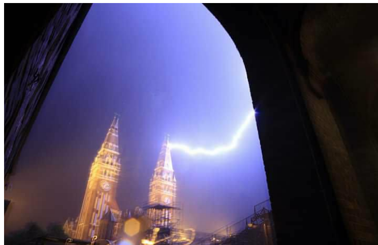
Figure 51: The lightning strike to roof-side of Szeged Cathedral in 2018 [99]
