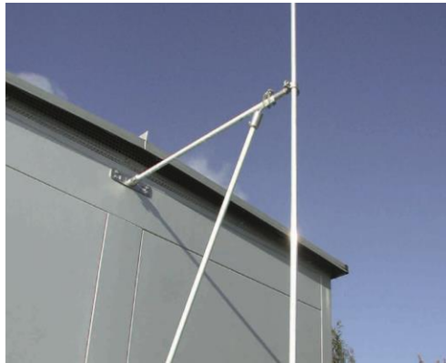
Figure 5: Arrestor held in a safety distance [16]
