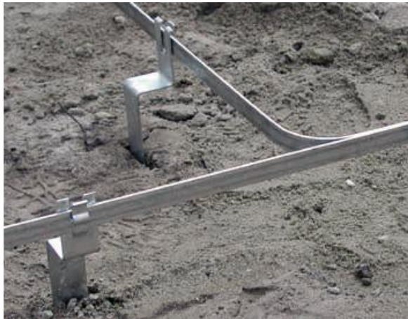
Figure 2: Foundation earth electrode [12]
